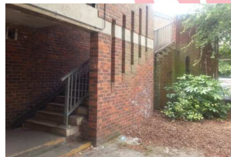
The existing footbridge to the north of the site
