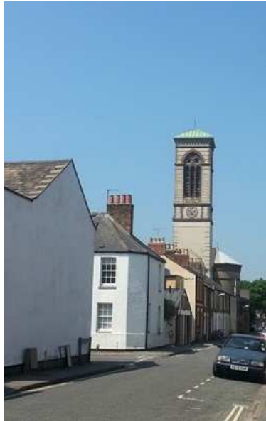
St Barnabas Church from Canal Street
