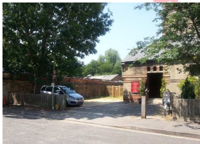
Wall at west end of the church to be removed
