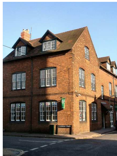
The existing Jericho Community Centre (photo courtesy of Isisbridge)
